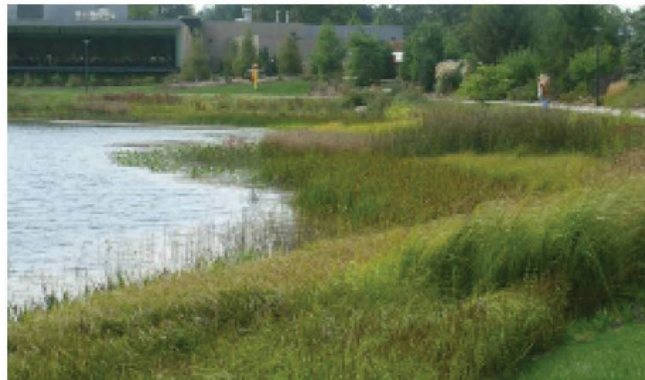
Image showing functional detention basin post-storm
